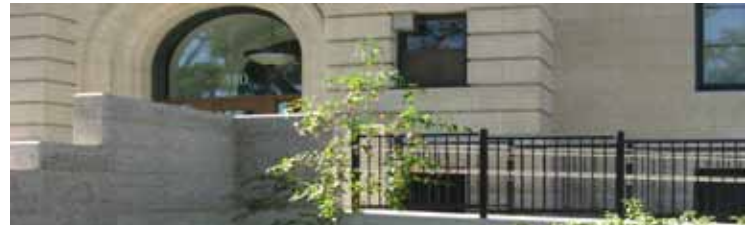
Winnipeg Archives Building
